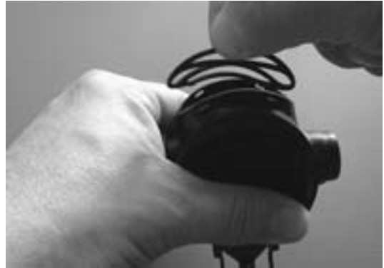
Fig. 8 – Exhaust Grille Installation
